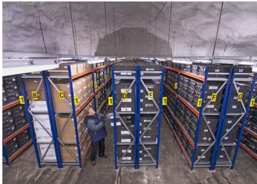
Concrete and plastic fiber on the seed vault's walls make them look like snow and ice. The real walls are dark-colored rock.
