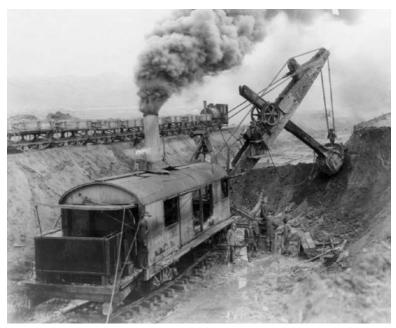
This is the kind of machine used 100 years ago to move earth. The machine was driven by steam. It had a water tank and a coal tank. The coal was used to heat up the water to produce the steam.
